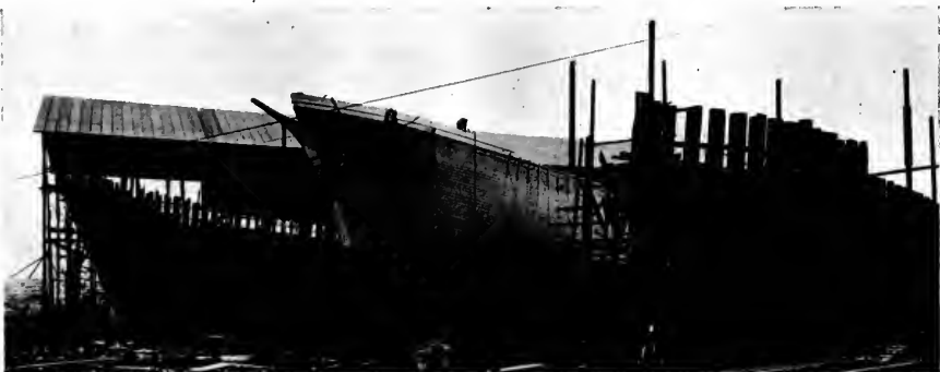
The building-ways at St. Helens, with one vessel ready for launching and two in frame.
